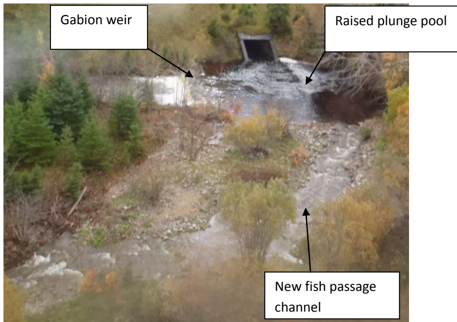
Fig 5 November 2012 photo of culvert pool and new channel under Fall flows.
